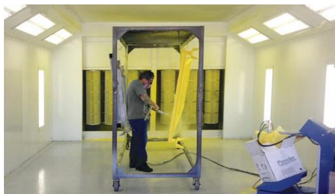
Custom Powder Recovery Booth with hip and sidewall lights
